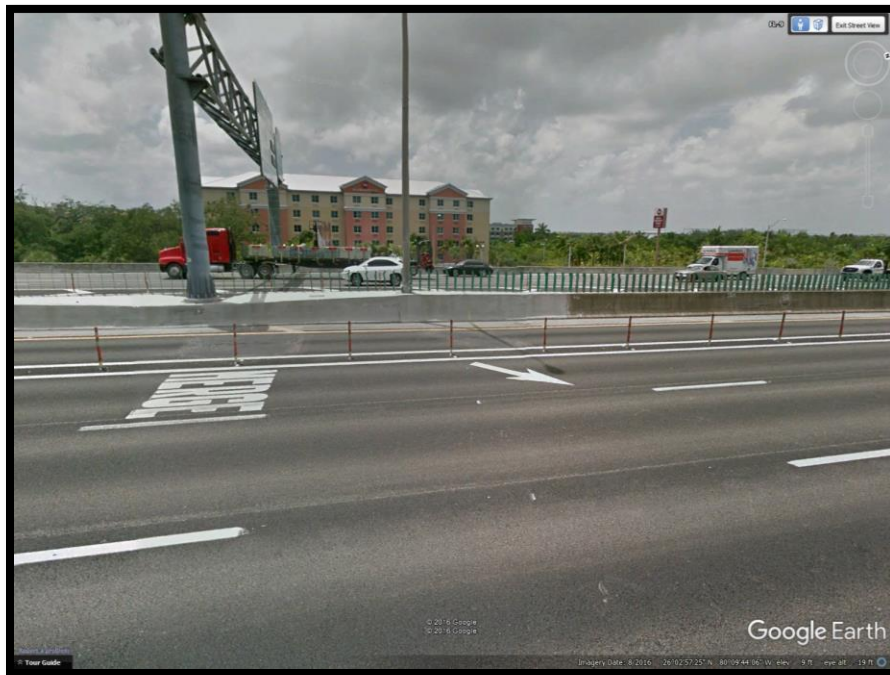
Figure 3.5 - Pavement Marking in the Exit of TML (Source: Google Earth)
