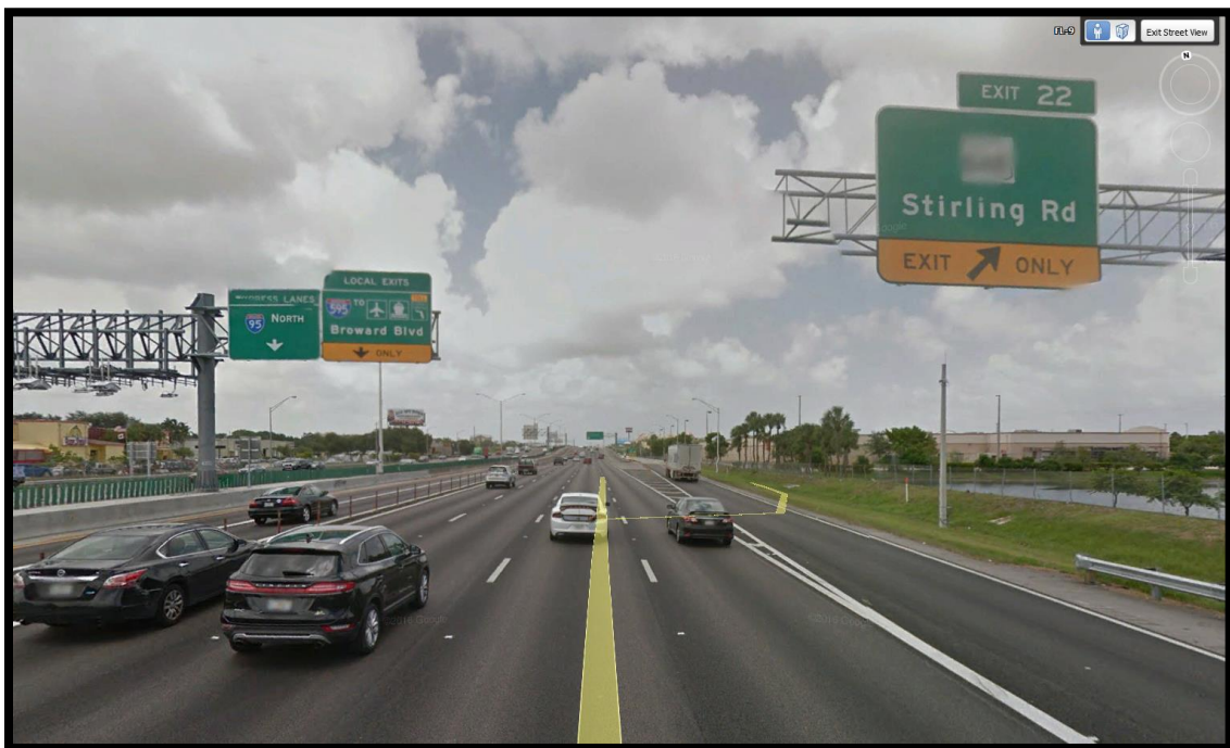
Figure 3.9 - Half Gantry Sign in the Exit of TML (Source: Google Earth)
